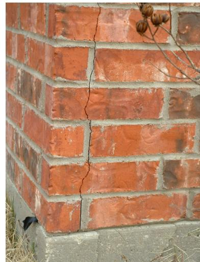
installed under warmer conditions, then under cooler conditions the brick will contract and creates a vertical crack within the brick and mortar starting immediately where the plastic membrane stops.
